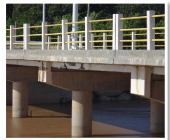
Flow gauging station under the Muinho Bridge over the Girául river
