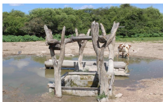
Figure 2: (a) Shallow Hand-dug well used for domestic purposes in the CEB of Namibia (Source: Hamutoko & McBenedict 2018); (b) examples of Deep hand-dug wells locally known as "Eendungu" (cylindrical-shaped hand-dug wells (Source: SASSCAL Task 007).
